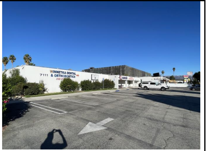
Photo 4: Asphalt paving on the east parking lot
