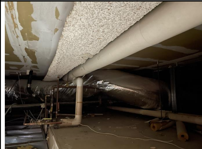
Photo 15: Non-ACM fireproofing on I-Beams above drop ceiling
